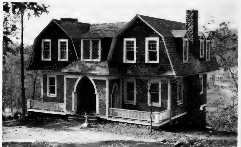
6—The Twin Gables in Gambrel Form are the Feature of the Exterior
